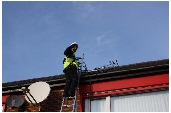
Placing roof ladder
