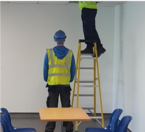
This is not safe
