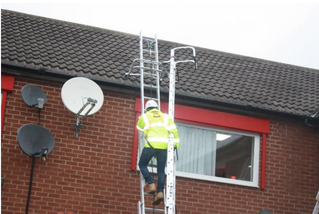
Carrying roof ladders up
