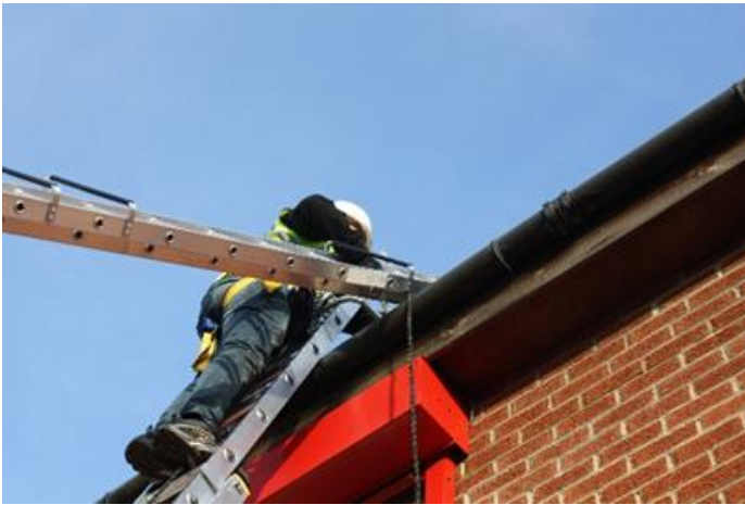
Lifting roof ladder 1
