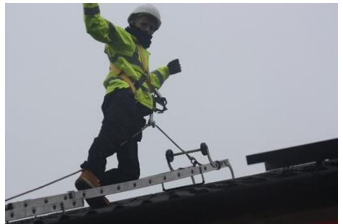
Top of roof ladder
