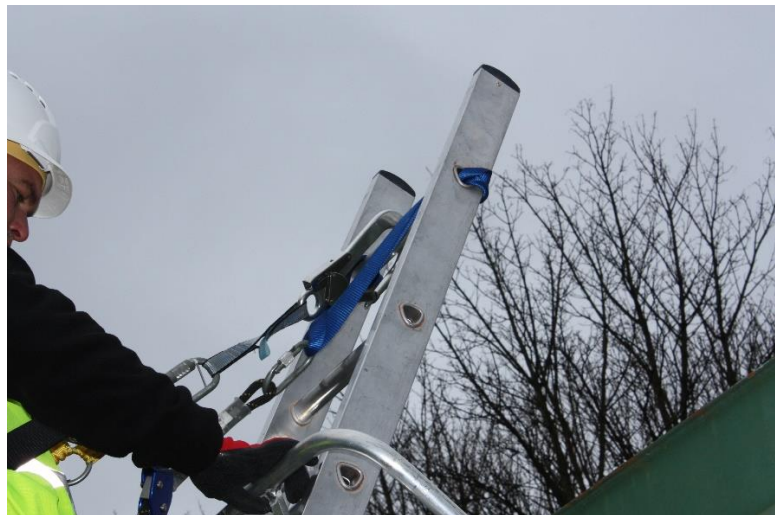
Cows tail attached to top rung of ladder
