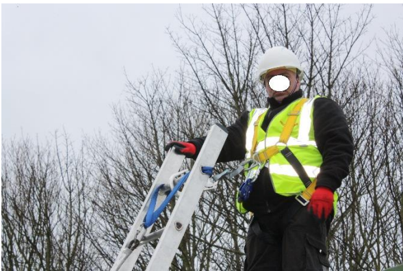
Engineer stood behind ladder attached with restraint lanyard
